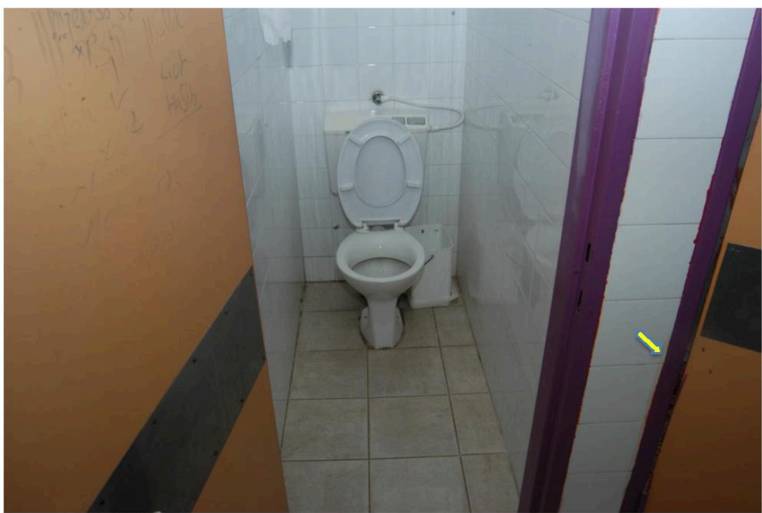
Figure 3 - Edges of the door's lintels of all the lavatory cells (Picture number 36). See arrows.
